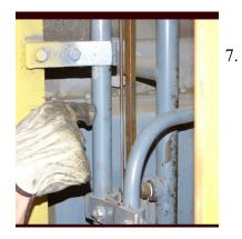
Check the water level sight glass to make sure there is water in the tank when the engine is cold. The water should be near the top of the radiator.
